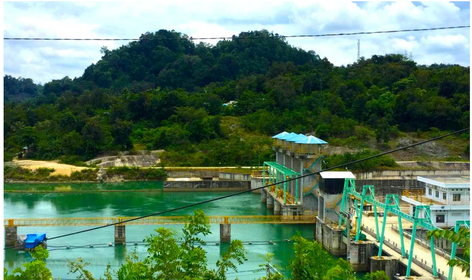
Poso Hydropower Plant Unit 2 in Sulewana area
